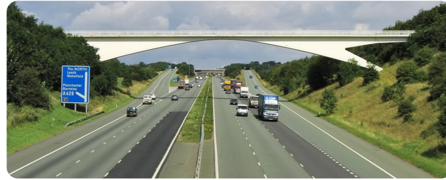
M1 motorway in Yorkshire
